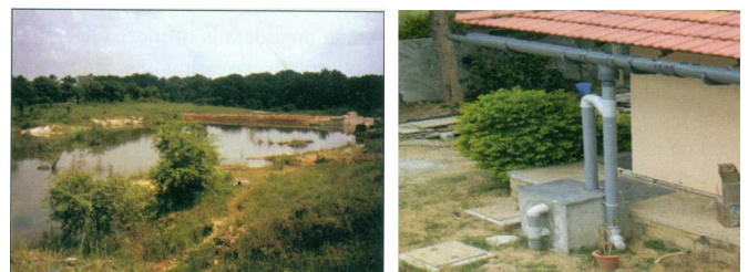
Fig.5. (a) RWH structure in Gyan Bharati Campus. (b) Roof Top Rain Water Harvesting in Bengaluru
